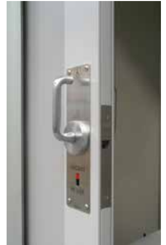
↑ CL100 Lavilock fitted to CS NewYorker glazed aluminium door.
