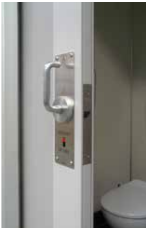
↑ CL100 LaviLock with standard lever handle fitted to CS NewYorker door.
